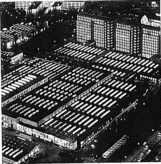
Switchgear Factory in Berlin, Germany
